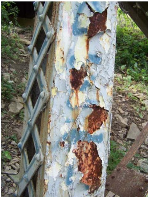
*Figure 1. Corroding support of a railroad bridge.*
