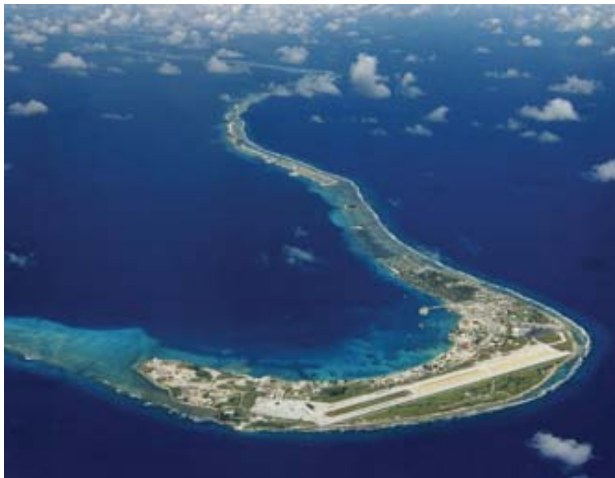
Aerial view of the Kwajalein Atoll in the Marshall Islands illustrating factors contributing to a high-corrosivity environment: tropical location, proximity of all locations on the island to the ocean, and low elevation providing no wind blocking. U.S. Army photo.
