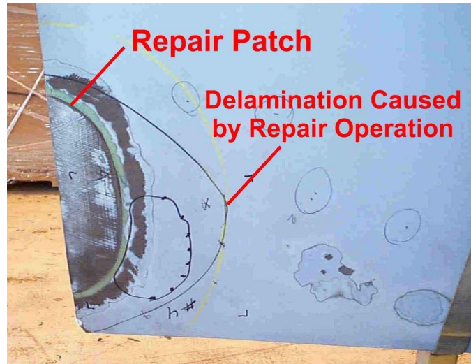
Figure 10. F/A-18 trailing edge flap following repair showing additional moisture-induced delamination during the repair operation.
